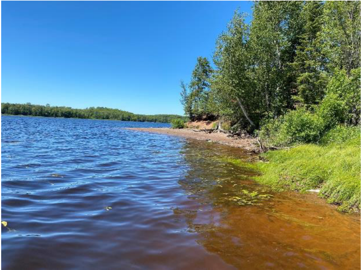
FIGURE 16. SITE #4 FROM THE 2022 GILE FLOWAGE SHORELINE STABILITY ASSESSMENT.
