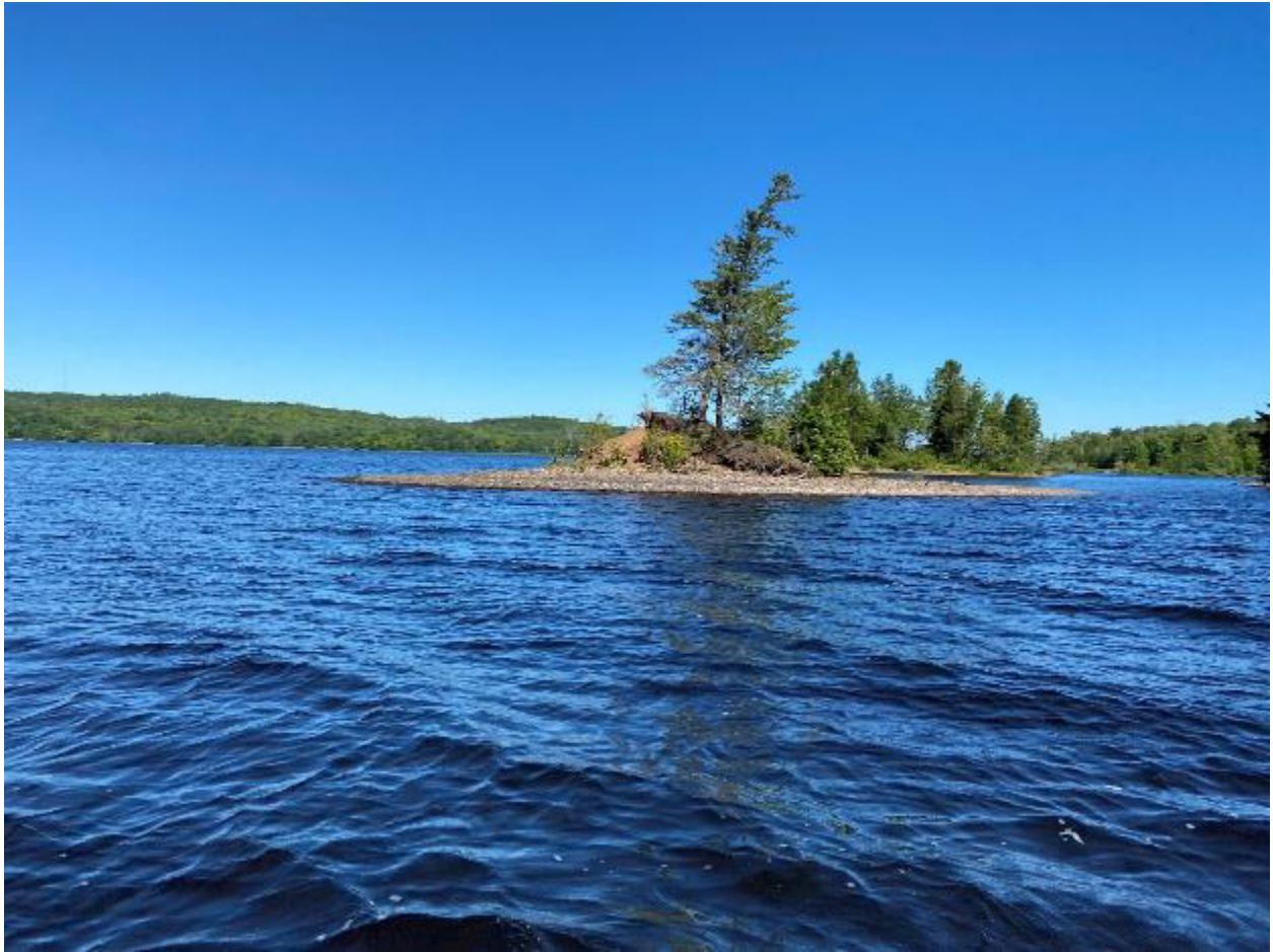
FIGURE 14. SITE #2 FROM THE 2022 GILE FLOWAGE SHORELINE STABILITY ASSESSMENT.
