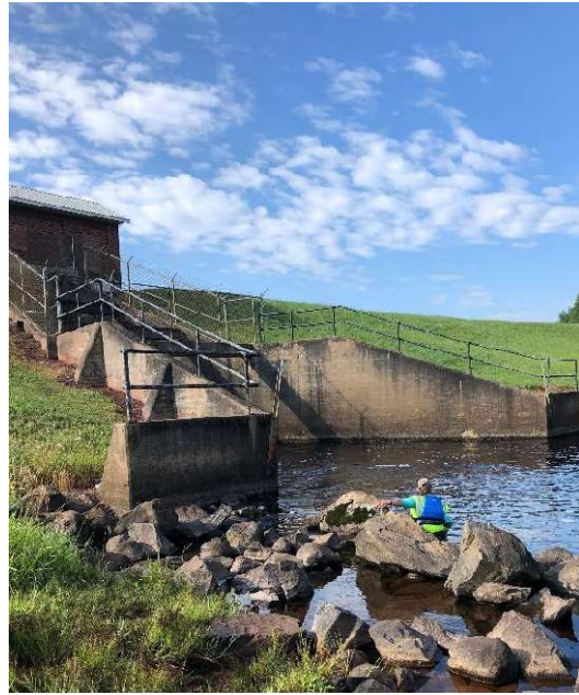
Gile tailwater sampling below the dam, 46.42594, - 90.22691 June 27, 2022
