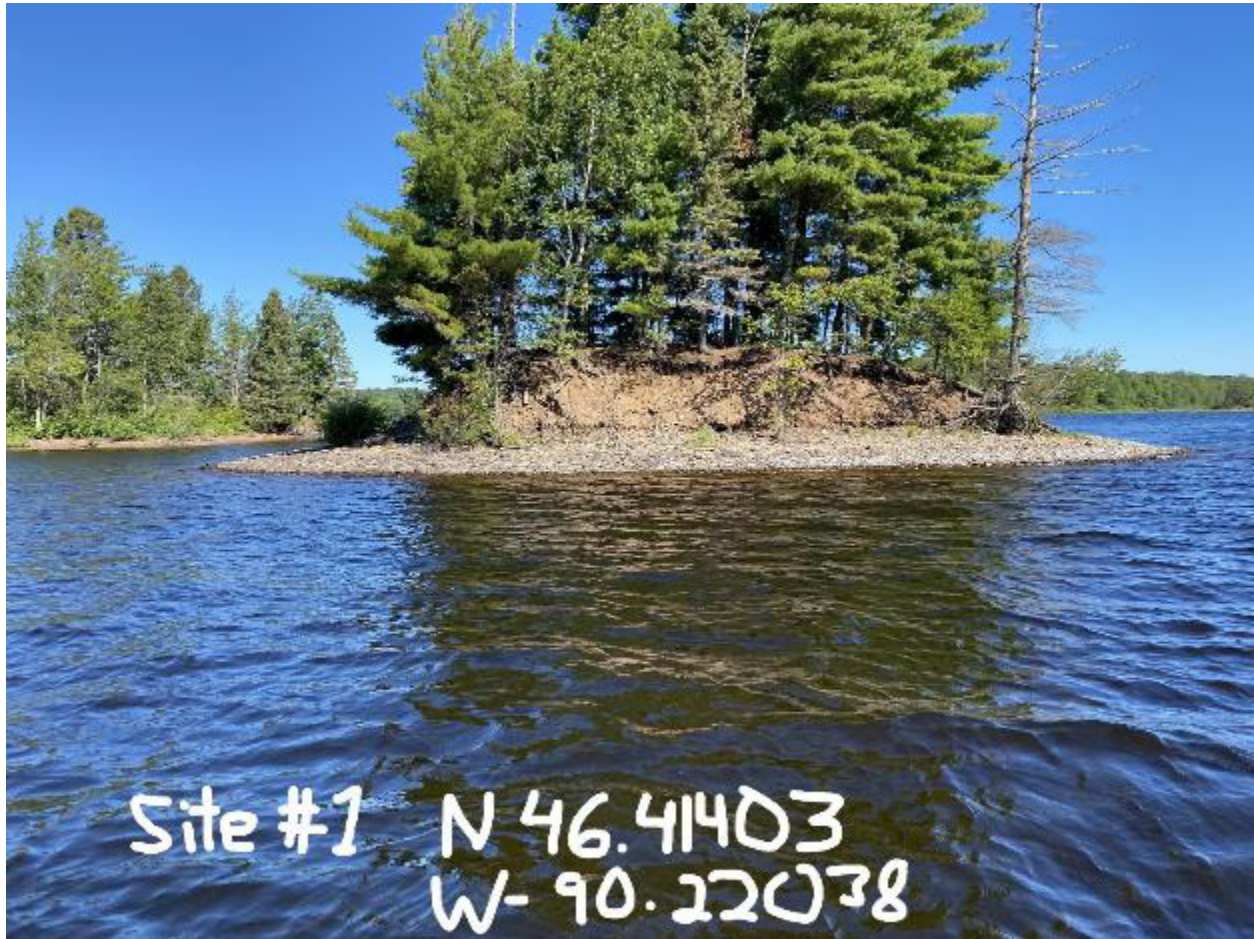
FIGURE 13. SITE #1 FROM THE 2022 GILE FLOWAGE SHORELINE STABILITY ASSESSMENT.
